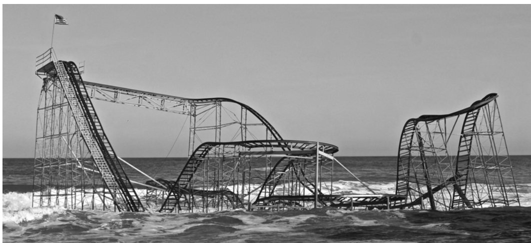
Source: The Jetstar roller coaster damaged by hurricane Sandy in October 2012, Seaside Heights, New Jersey, published by Flickr.com, © 2013.
